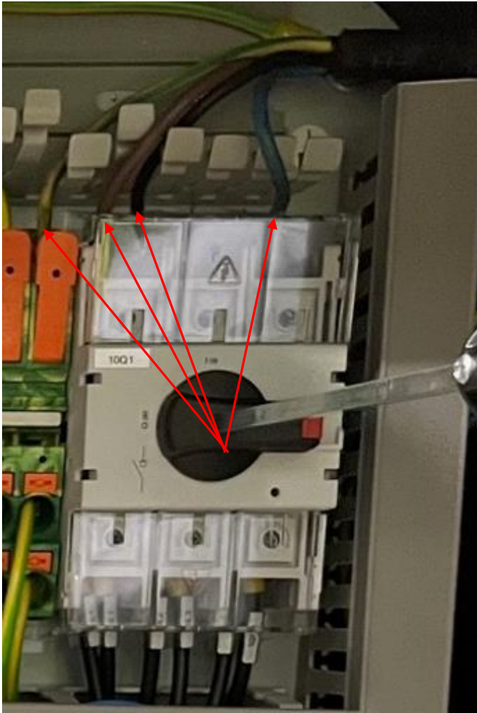
Power connections to the FRAMECAD TF550H
