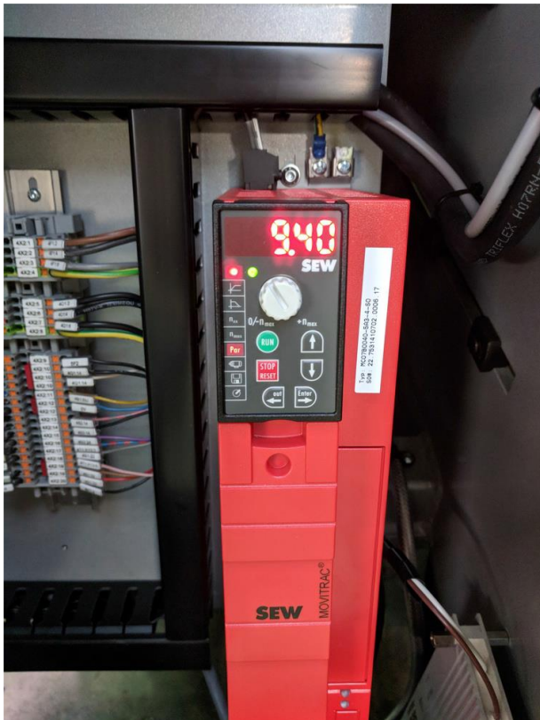
Fig. 3 P20 (voltage feedback) display showing 9.4V from inclinometer
